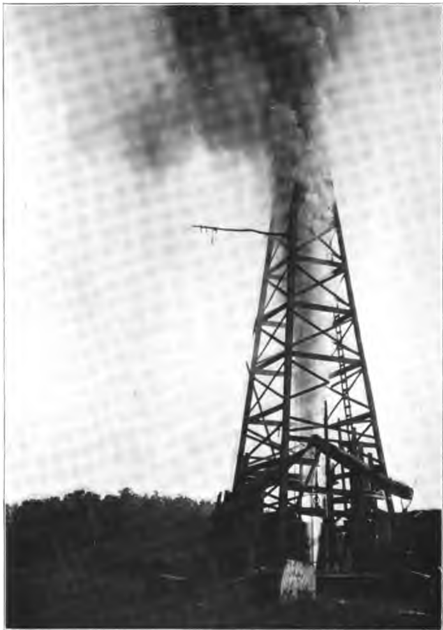
PLATE XVI.—Effect of Shot on the Paugh gas well (704) in Fifth sand, located two miles S. E. of Byron. Dry sand loosened by the Shot is being blown out with the gas.
